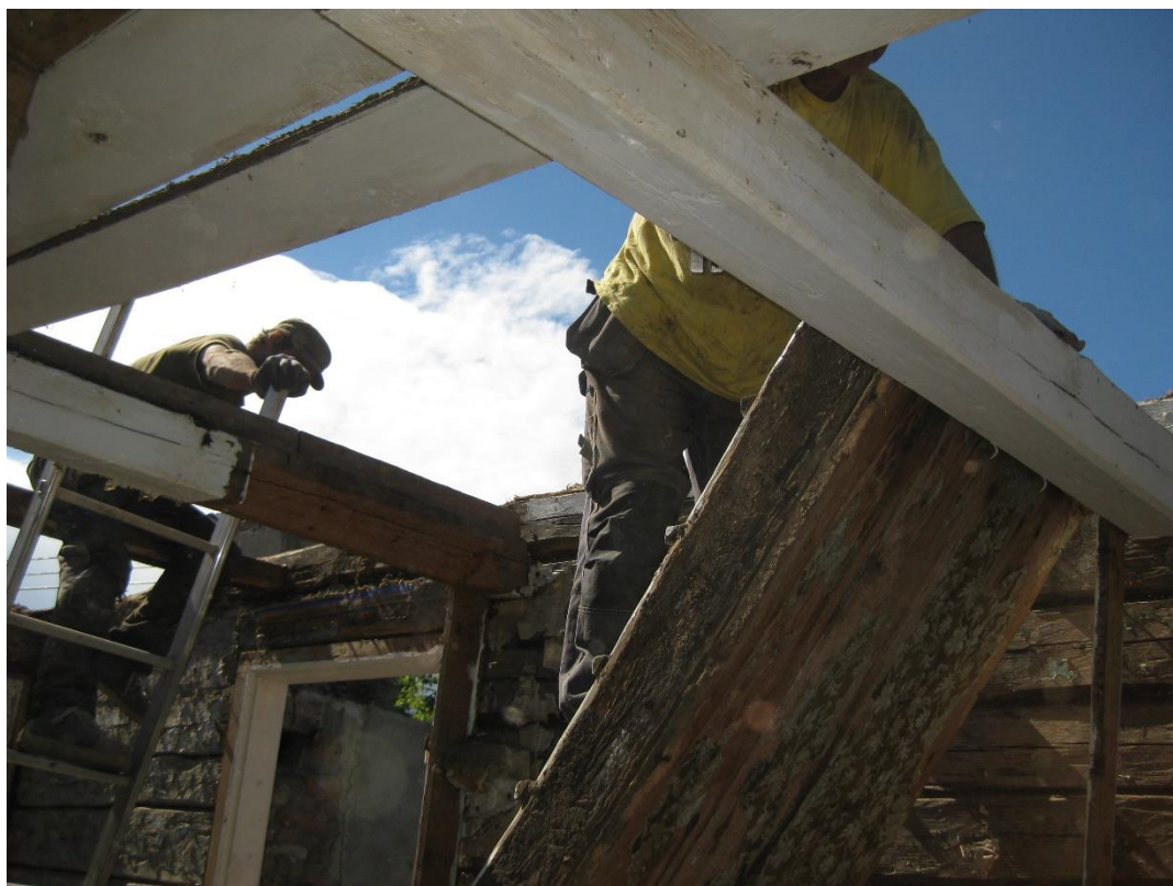
Stockarna monteras ner.
